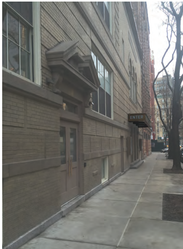
EXISTING – VIEWING LOOKING WEST
