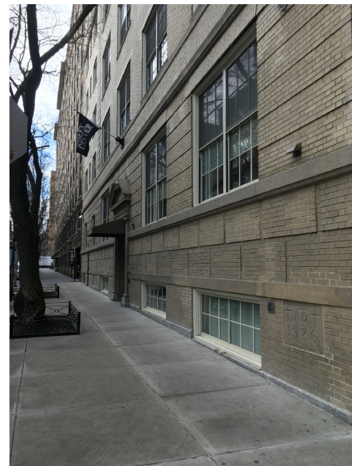
3 VIEW OF ELIZABETH STREET ENTRANCE
